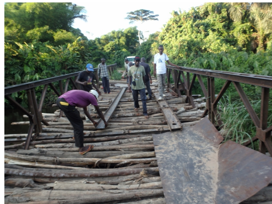
Figure 2.8: “Distribution team sets an iron ledge over unstable bridge to help people cross by foot.” Photo and caption courtesy of AMF.
